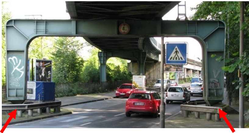
Tilted bearings activate the arch thrust!
